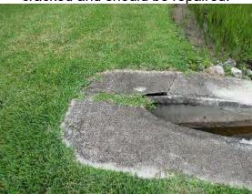
c. Erosion: Runoff from Building B is causing erosion on the west bank of lake 1.
